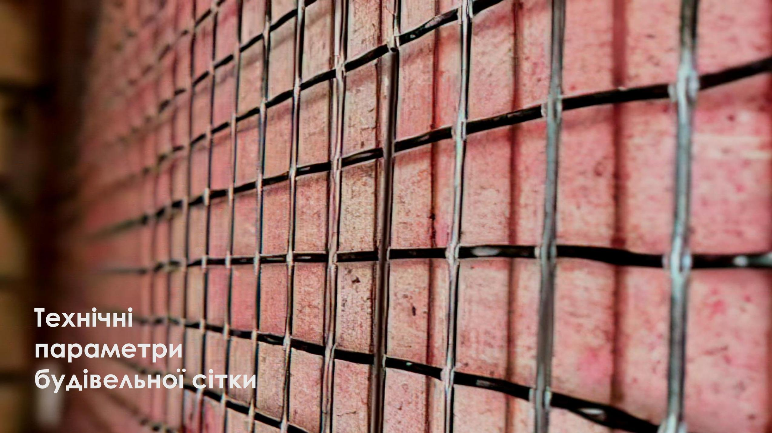
A close-up photograph of a red brick wall. A dark metal mesh, likely galvanized steel, is overlaid on the bricks. The mesh consists of a grid of vertical and horizontal wires, with the intersections welded together. The bricks are arranged in a standard running bond pattern. The lighting is somewhat dim, highlighting the texture of the bricks and the metallic sheen of the mesh.
